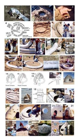
Figure 2 The building process of Superadobe Source: www.calearth.org
